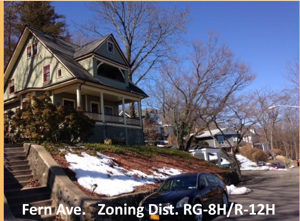
View of S.N. from above on Fern Ave
