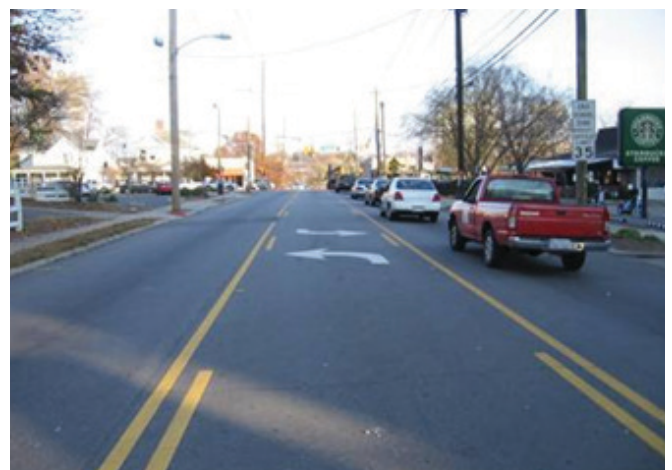
Figure 52. An example of a two-way left-turn lane.
