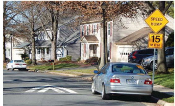
Figure 48. An example of a low-speed residential speed hump.
