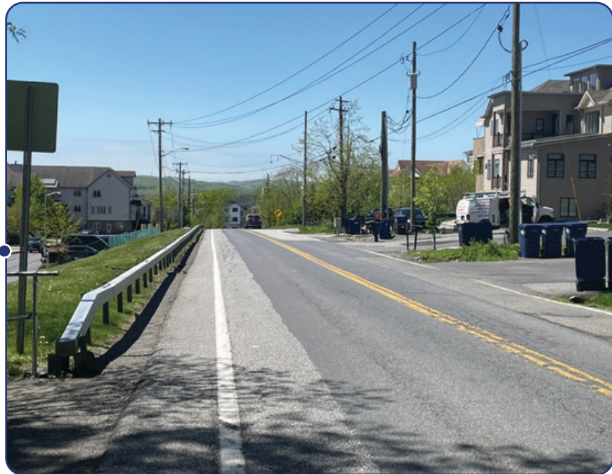
Figure 20. Seven Springs Mountain Rd
