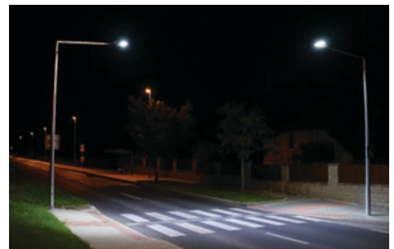
Figure 42. An example of a well-lit pedestrian crossing.
