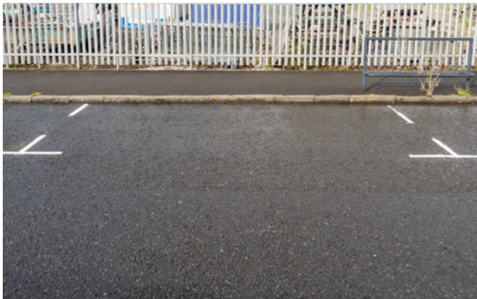
Figure 53. Parallel parking road markings
