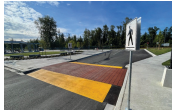
Figure 41. An example of a raised crosswalk.
