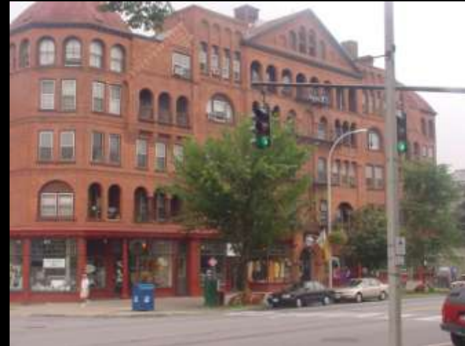
Re-use of established architectural icons in a downtown environment.
